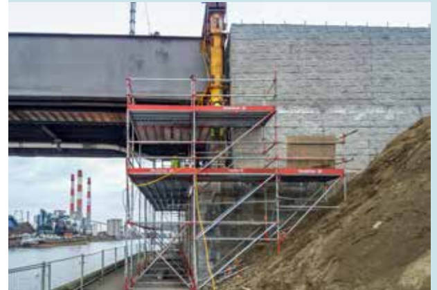
KOLENHAVEN | GENK, BELGIUM
