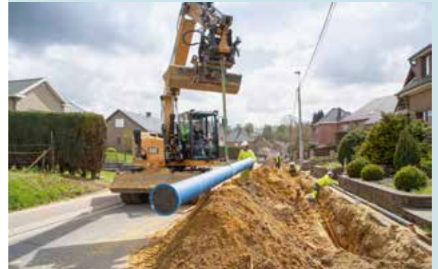
LAYING SUPPLY PIPING | TERVUREN, BELGIUM
